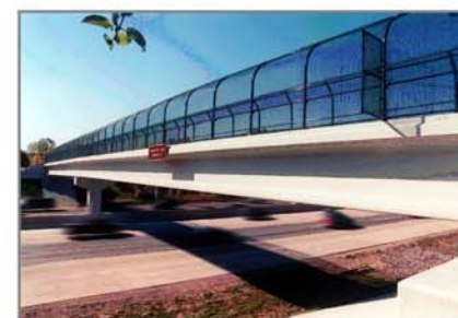
Pedestrian bridge spanning I-75
